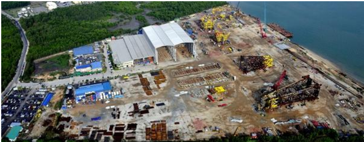
Figure 1: Pulau Indah fabrication yard
